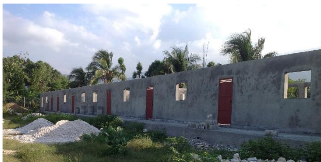
Construction as of April 2016
